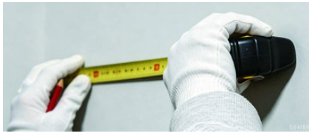
Measure before cutting
